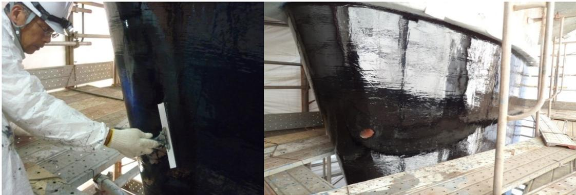
First coat of Belzona 2141 applied      Application completed
