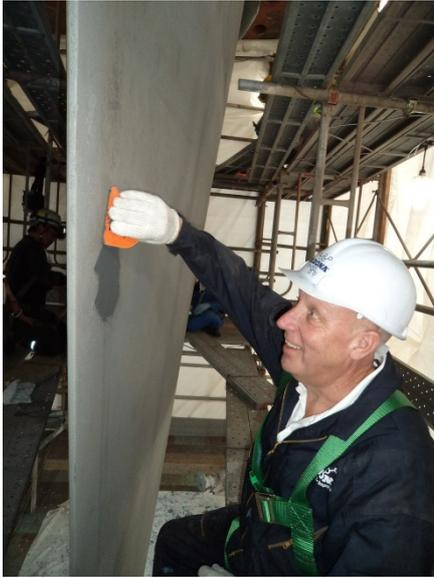
Pit filling with Belzona 1311
