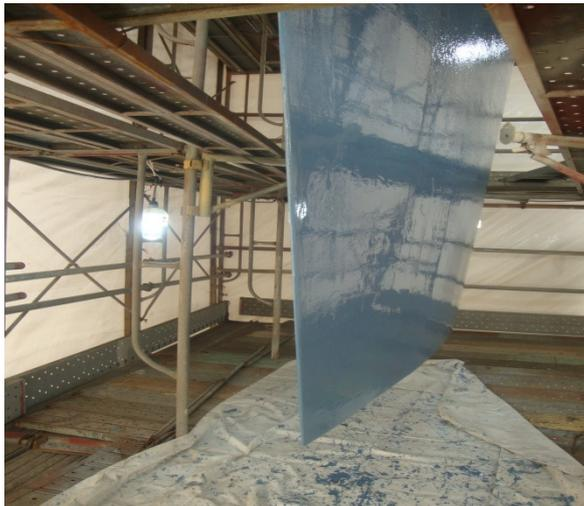
Anti-corrosion coating Belzona 1341
